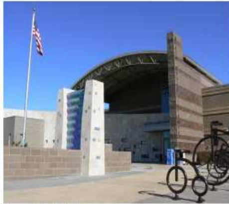
Queen Creek Library, Arizona
